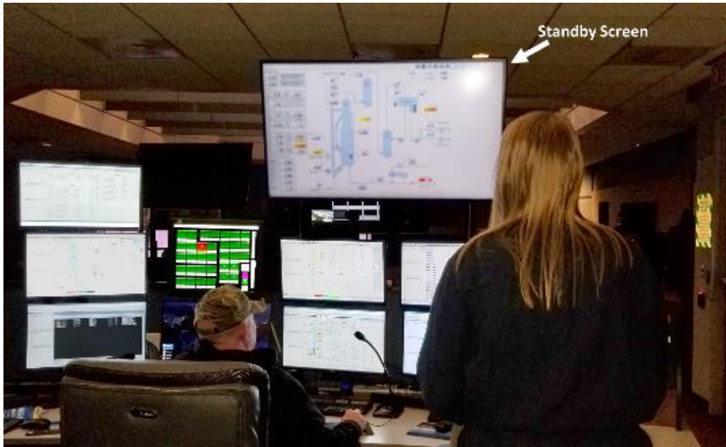
Figure 1. Simplified DCS screen for FCC standby operation at console
