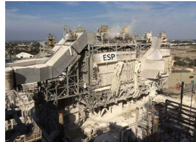
Torrance 2015 Incident: ESP Damage CSB Investigation Report, Figure 18
