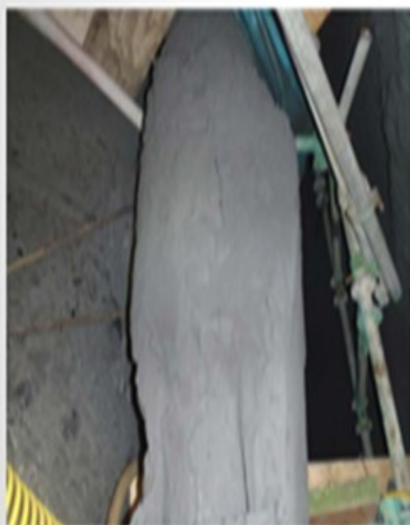
Deposits on Reactor Cyclone Dipleg
