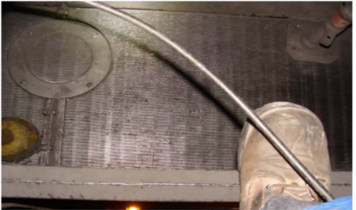
Reactor Catalyst Support Deck – After CO 2 Blasting
