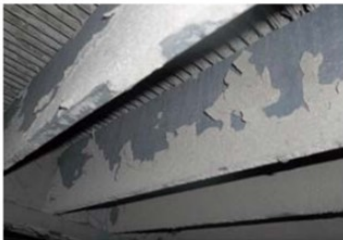
Reactor Catalyst Support Deck – Underside Scale
