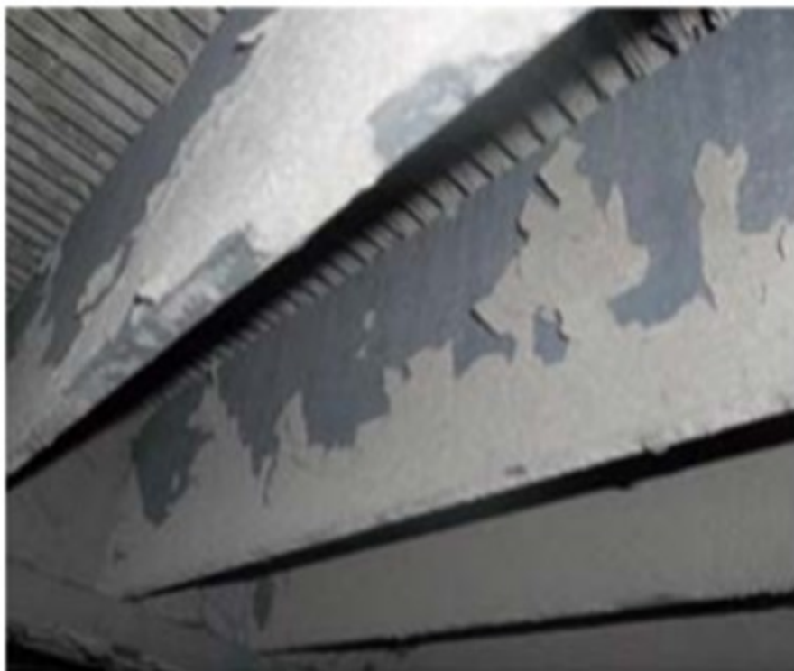
Reactor Catalyst Support Deck – Underside Scale
