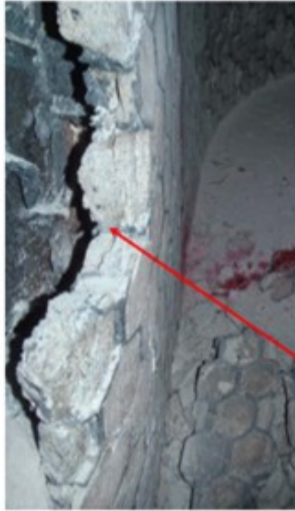
Alternate refractory lining failure due to under-lining corrosion on exterior of regenerator cyclone diplegs.
