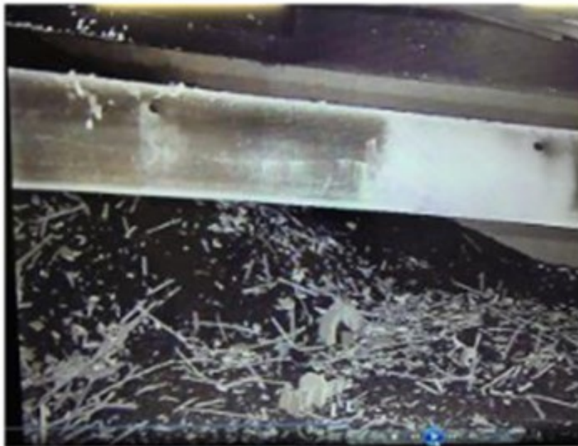
Figure 3. Catalyst found on Intubed Redistribution Tray
