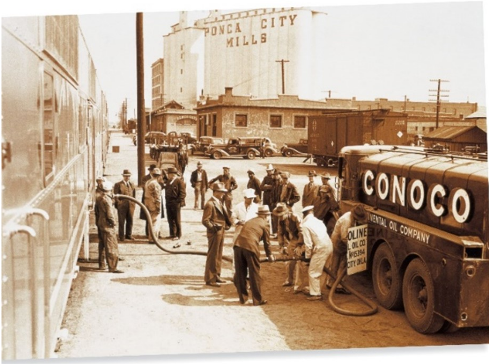
Ponca City Refinery, 1939. Credit: Phillips 66 Historical Archives
